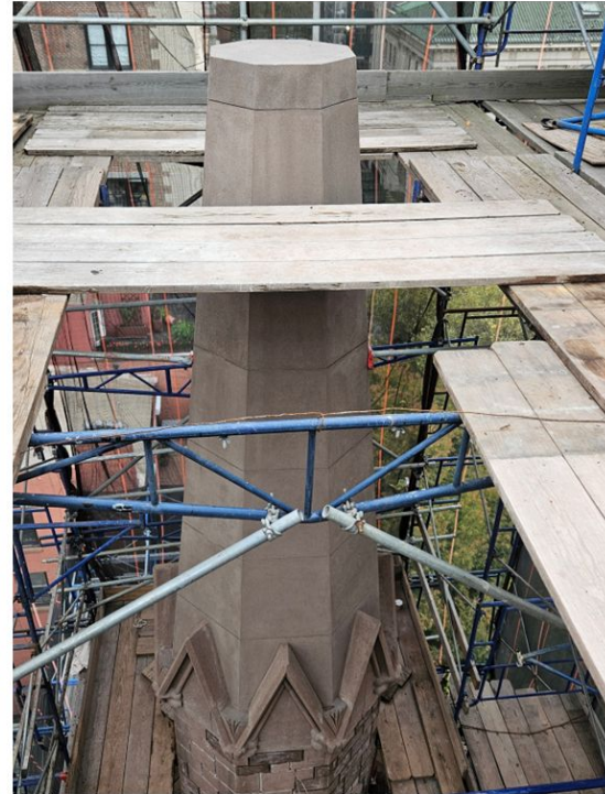
Current State: brownstone repaired and ready to receive fiberglass.
